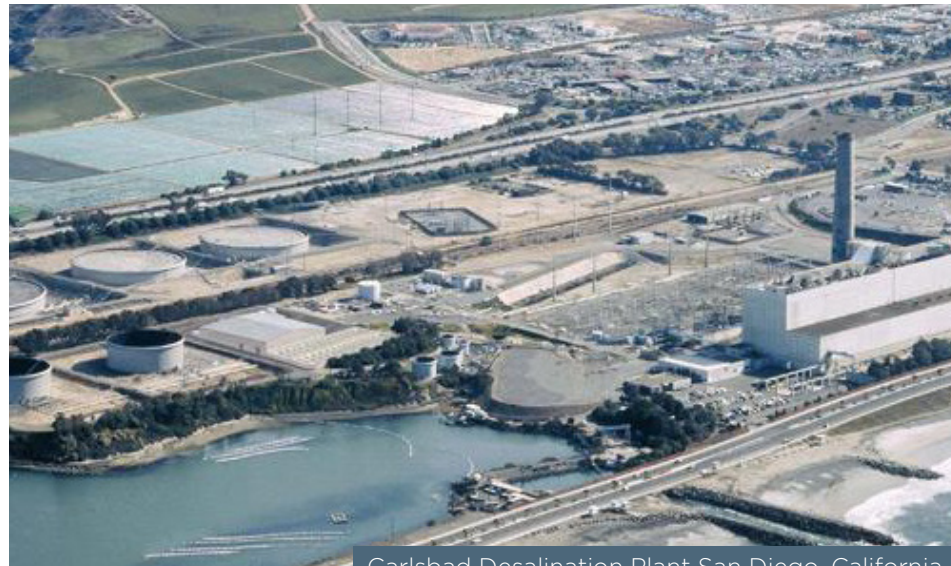
Carlsbad Desalination Plant San Diego, California
