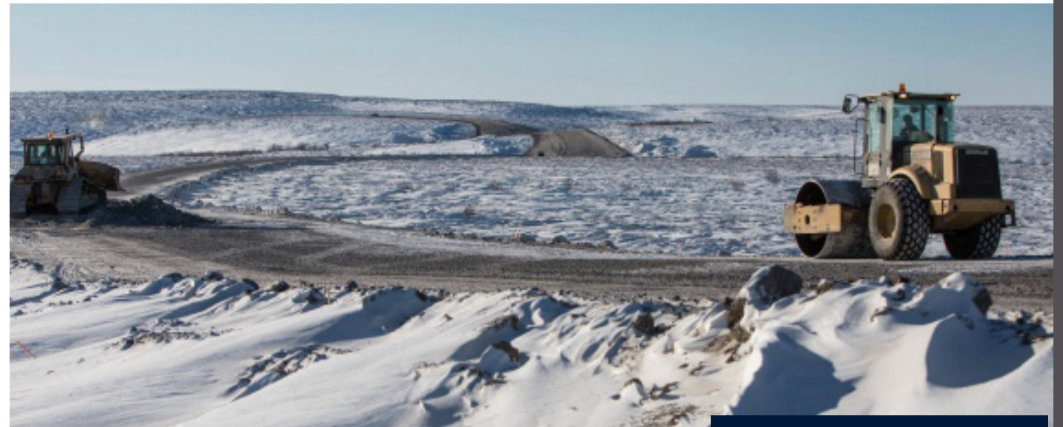
Crews work on the Tuktoyaktuk end of the Inuvik to Tuk all-weather road. Credit: James MacKenzie, Dept of Transportation (Transport Canada)
